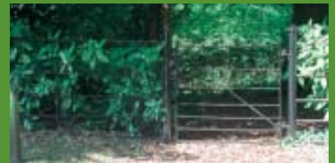
Iron gate and matching railings – The Old Rectory.
