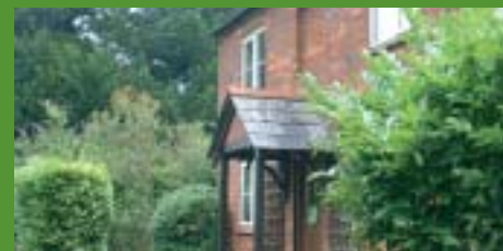
Porch at Laurel Cottage – constructed in proportion to the building.
