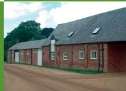
Old stables at Manor Farm adapted to office use.
